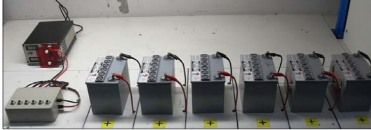
Figure 16: Charger Station Reference Layout 2 (Front View)
