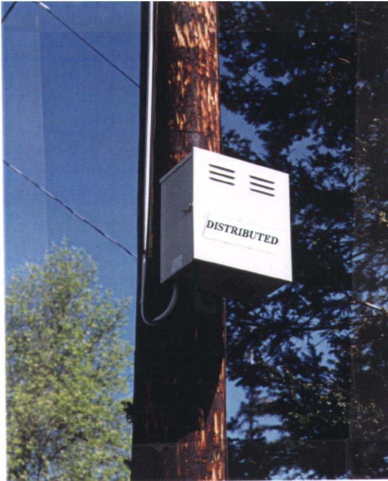
**Photo 2** Pole mounted distributed standby power supply
